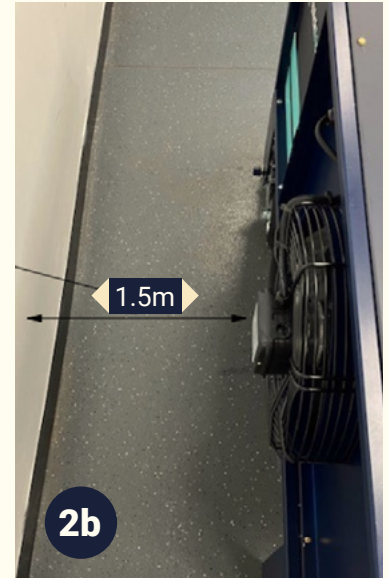
Minimum 1.5 metres distance from Quickfridge to nearest object e.g. wall (Unit blow side)
