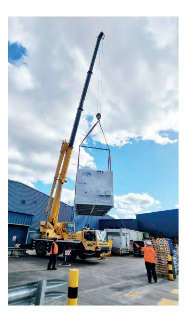
The high quality transcritical pack features "Plug 'n Cool" design, meaning that installation required only a mains supply and connection of the suction and liquid pipework to the system. Using a 4-fan vertical discharge condenser and four Bitzer 4FTE-30K compressors provided an all-in-one solution.
